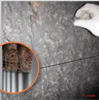
Ash sticks to the surface of boiler walls, super heaters, reheaters, and economizers.
